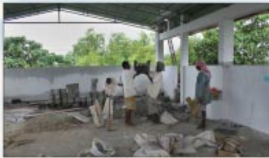
Kindly pray and help for the 24 hours prayer tower construction work to be completed.
