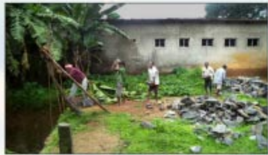
Our Vishwasada Mane's drainage work is in progress.
