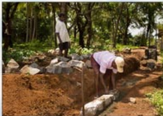
Kindly pray and help for the boundary wall of the new place and construction work to be completed.
